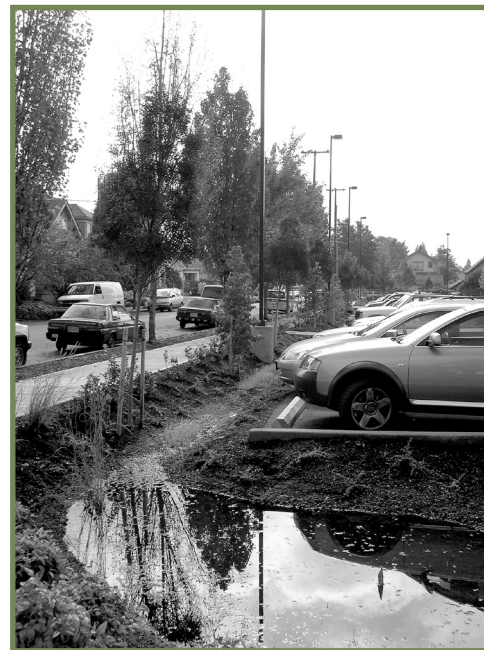
Stormwater swale, recently planted
